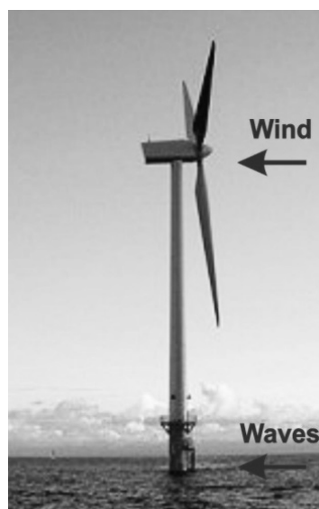
Figure 1: Offshore Wind energy plant under unknown dynamic loads from wind and waves.
